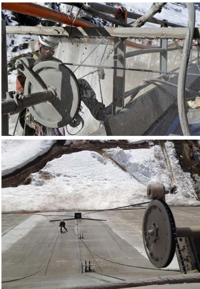
Figure 80: Travaux de sciage.
