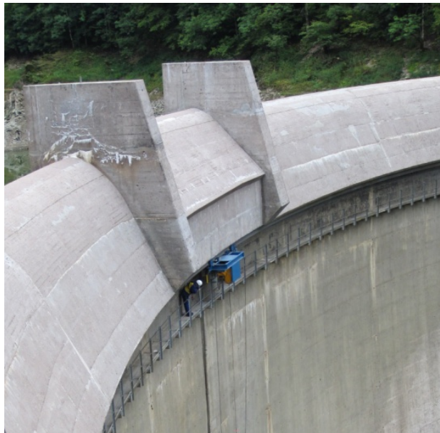
Figure 54: Aspect des murs guideaux: fissuration horizontale.
