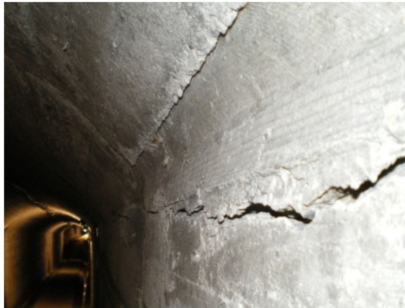
Figure 77: Galerie de pied – fissuration.
