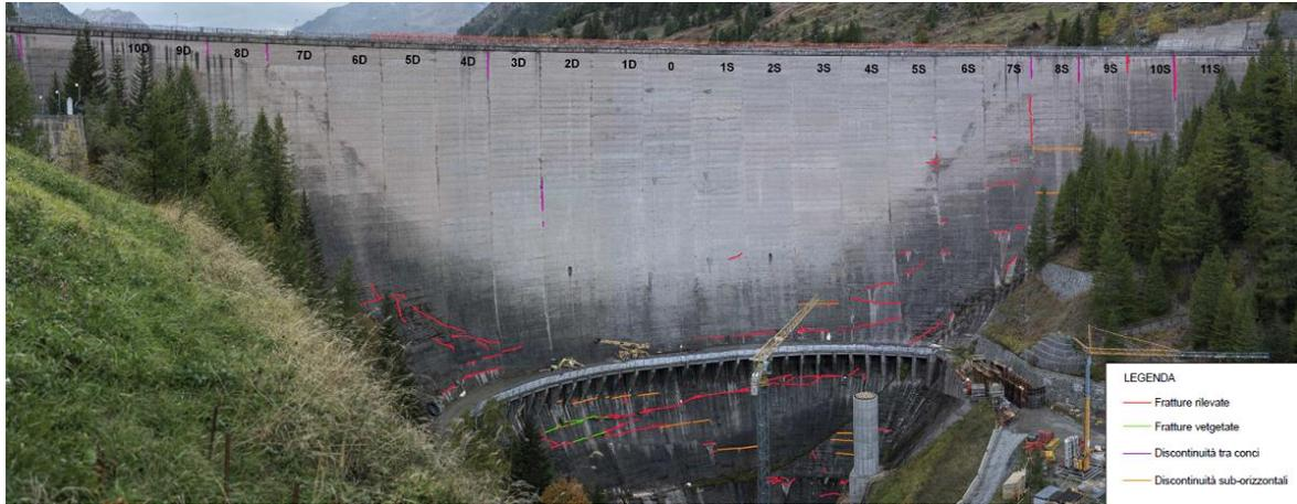
Fig. 4: The dam was observed to deflect upstream with cracks (depicted in red) appearing on the downstream face and openings of some upstream vertical joints
